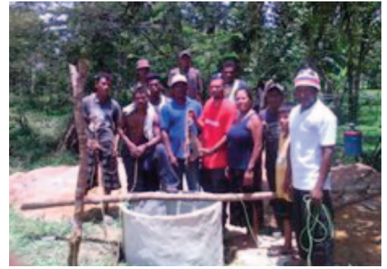
A new well nearly finished
