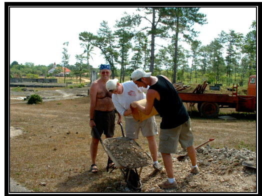
Ralph Gabarro, Seth Gabarro, and Manuel LeBlanc making cement blocks for the new operating room.
